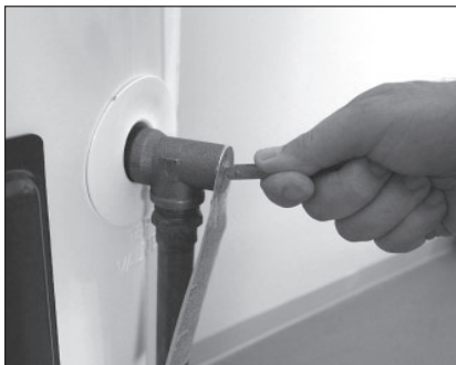
Figure 40 - T&P Relief Valve
